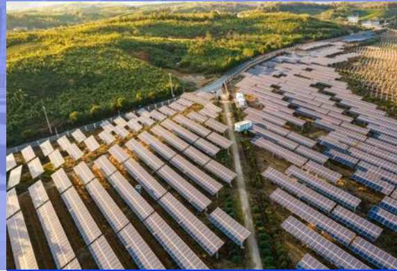
Agriculture-Complementary Solar Power Station
