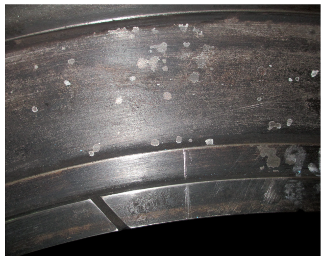
Fig. 2: Installation in the original position according to the markings
