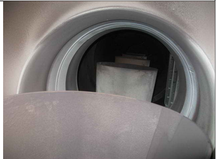
Inspection area No. 6: take photo of exh. receiver. Comment:
