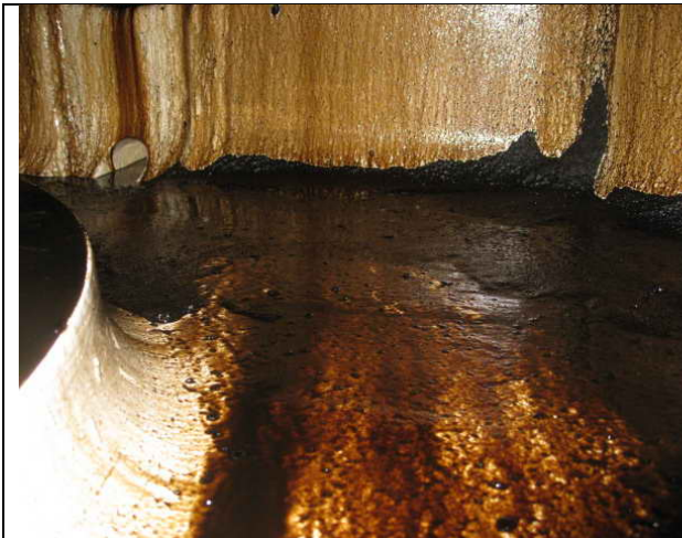
Inspection area No. 3: take photo of drain line from the buffer spaces. Comment:
