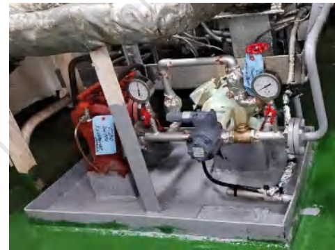
Pump Station Modification
