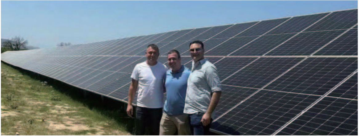
20MW PV Power Station Project
