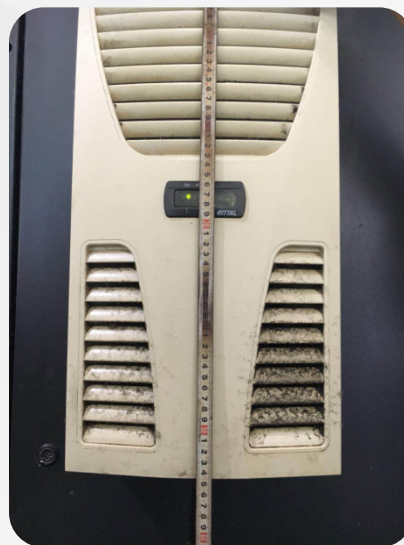
2-The length of the AC to be replaced.
